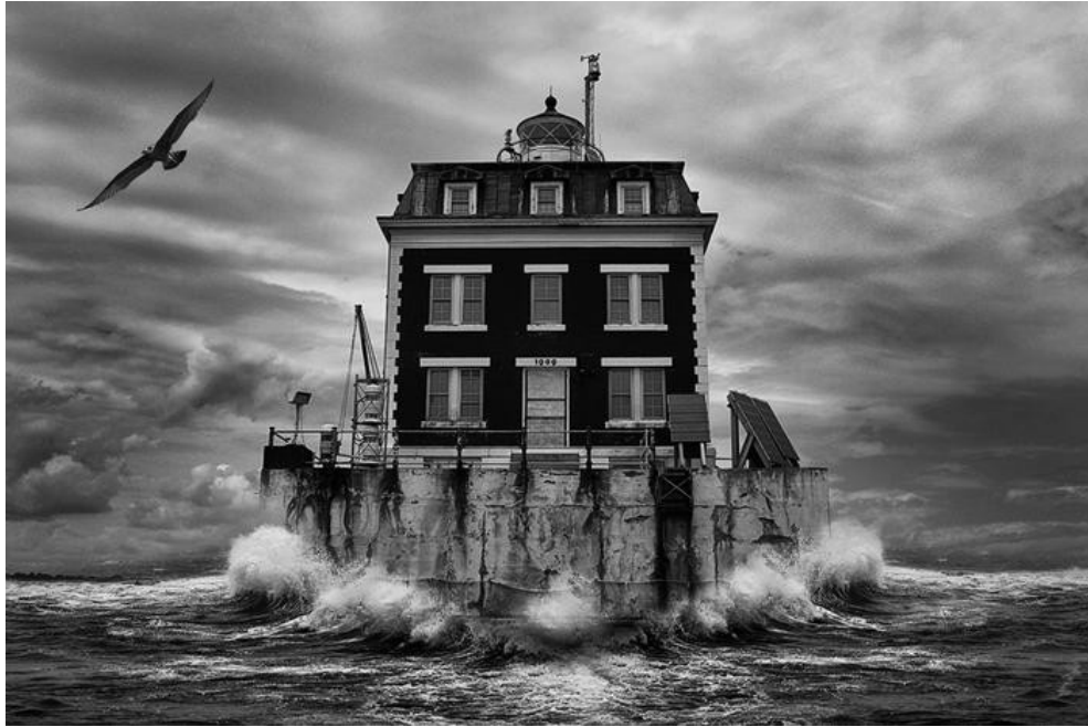
Photo Courtesy of http://www.ledgelighthouse.org/deterioration.html
