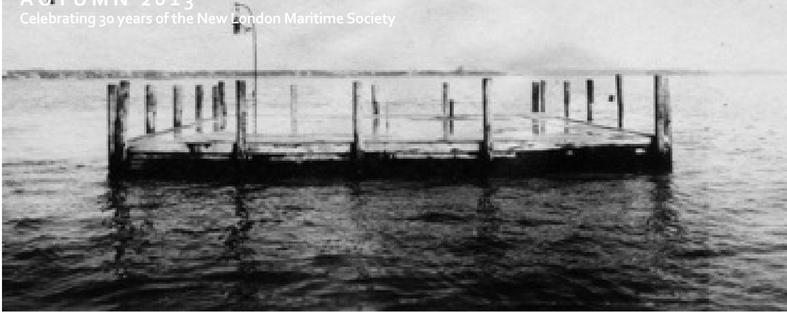
Above: The foundation of New London Ledge Lighthouse, ca. 1908. Photograph courtesy the Henry L. Ferguson Museum Collection.
